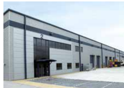
Network Oxford The first phase of Rego Oxford's Network Oxford scheme was completed with VSL's letting to Speedy Hire who joined Travis Perkins at a new trade destination.
