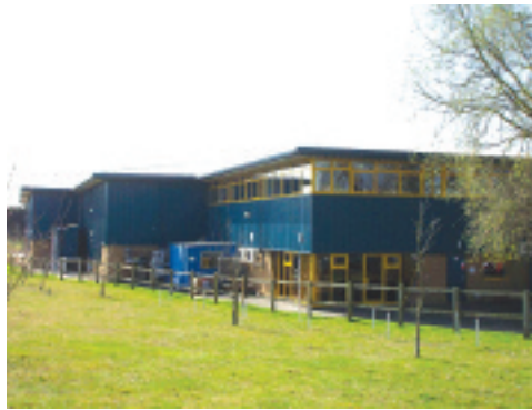
Enterprise House, Standlake Let by VSL to Pizza Express plc. A purpose-built food production unit
