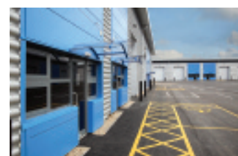
Nimrod, Witney. A small unit industrial scheme of 40,000 sq ft in Witney by Abacus Developments. 5 units sold prior to practical completion
