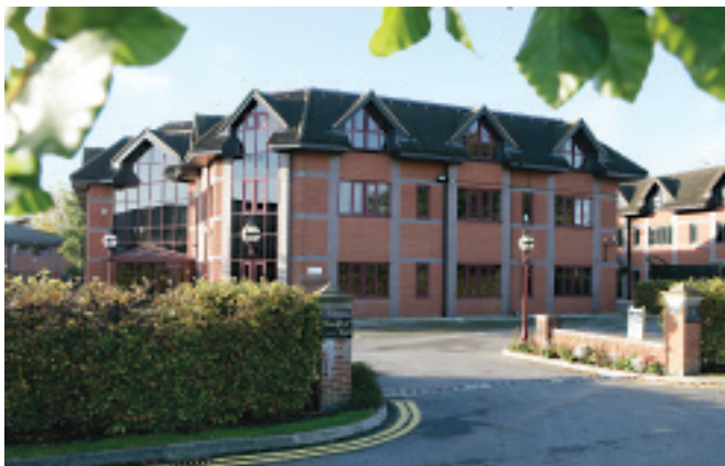
East Point Business Park, Oxford Road.
