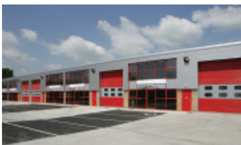
Nuffield Centrum, Abingdon. Refurbished units by ING. Lettings in 2007 included Sally Hair & Beauty, BSS, Southern Brick & Tile and Leeches Printers. Rents achieved between £6.50 and £8.50 psf
