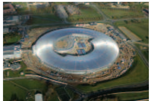
The Diamond Light Source project under construction.
