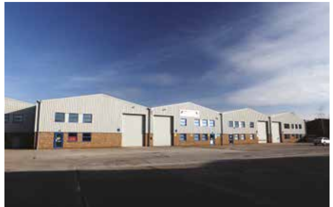
Units 12-20 Avenue One, Station Lane, Witney On behalf of Thames Water Pension Fund VSL leased 12,000 sq ft of warehouse space to Howdens Joinery on Witney's busiest industrial estate and sold 11,000 sq ft to Gomaco.
